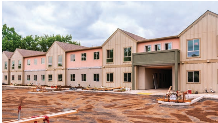
OAK PARK SENIOR APARTMENTS under construction PHOTO CREDIT: DOMUS DEVELOPMENT
